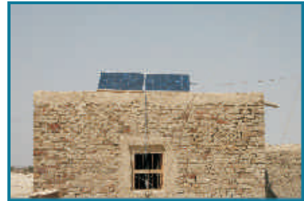
Solar Panel on top of the roof
