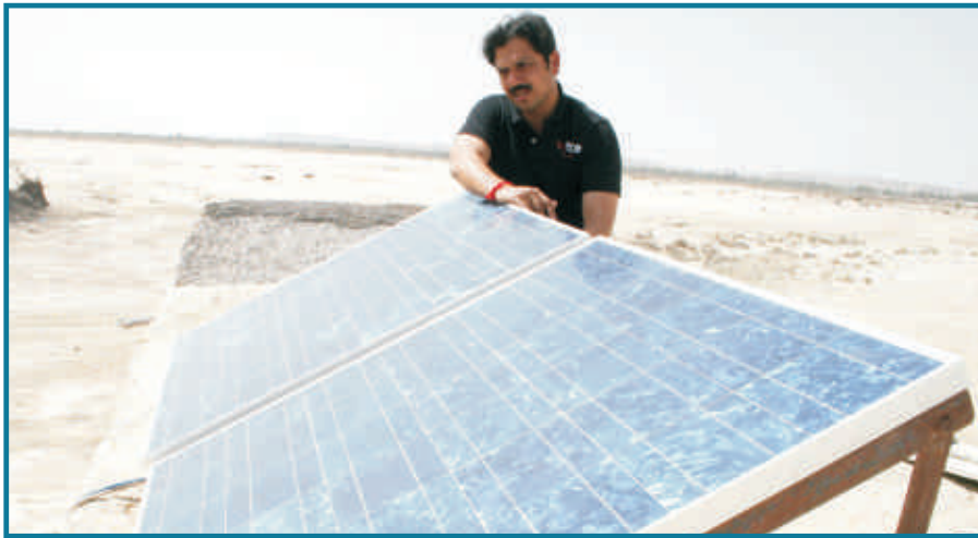
Solar Panel is being installed
